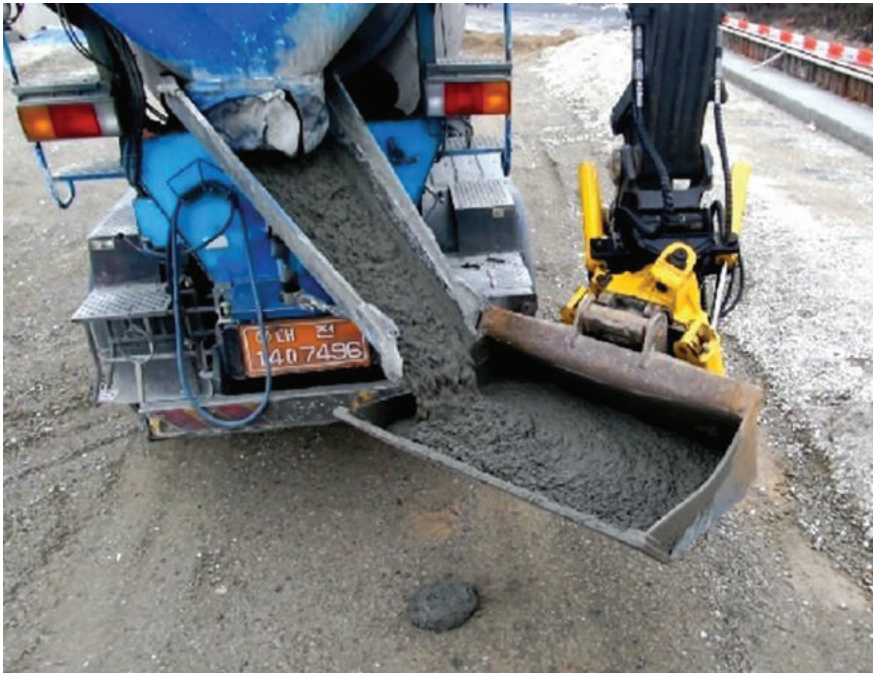
Placing ready-mixed concrete
